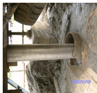
Installation Of Screen To The Hole
