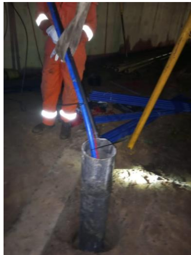
Anode installation in progress.... [Cathodic protection]
