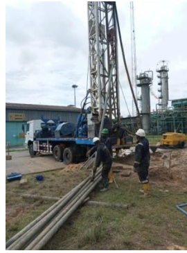
Pulling Out of Drilling Pipe...
