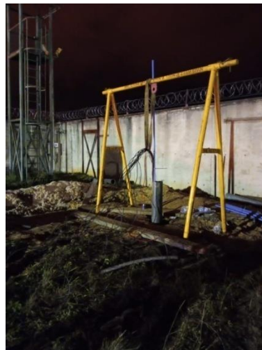
Anode installation in progress.... [Cathodic protection]
