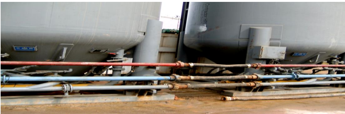
Sandblasting and painting of the silo tank.
