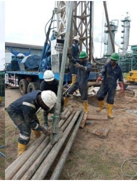
Pulling Out of Drilling Pipe...
