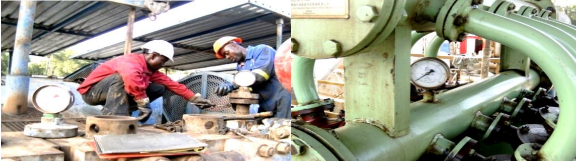
...Installing pressure guage in process by Dee.p Resournces personnel...
