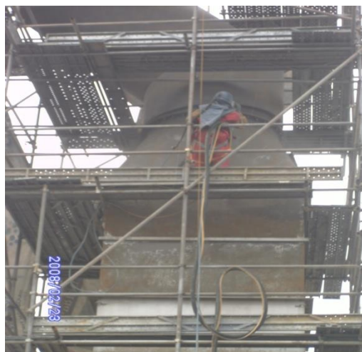
Erecting Of Scaffolding In Spdc I.A @ Rumuomasi PHC. / Sand Blasting Of Heat Exhaust In Spdc I.A Gas Turbine.
