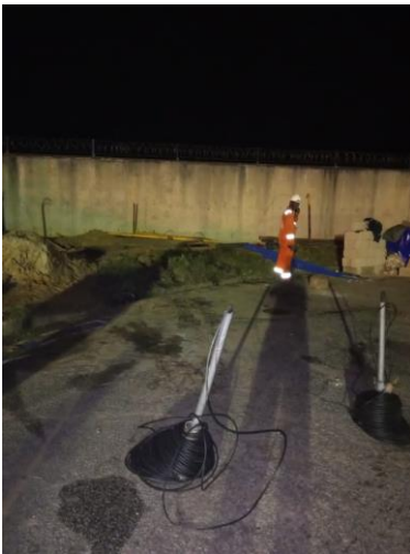
Anode installation in progress.... [Cathodic protection]
