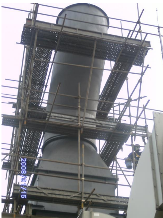
Primer Of Gas Turbine @ Spdc I.A Rumuomasi In PHC. / Painting Of Heat Exhaust Of Gas Turbine In Spdc I.A Rumuomasi In PHC.
