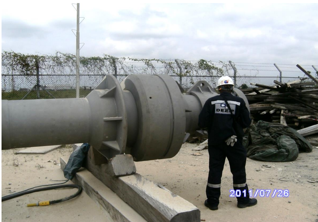
Supervisor Inspecting the Blasting Surfaces.
