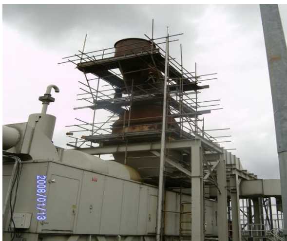
Erecting Of Scaffolding In Spdc I.A @ Rumuomasi PHC. / Sand Blasting Of Heat Exhaust In Spdc I.A Gas Turbine.
